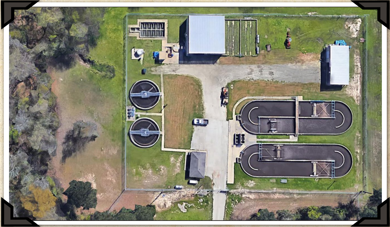
NORTH ANGELINA COUNTY REGIONAL WASTEWATER FACILITY GOOGLE EARTH AERIAL IMAGERY
