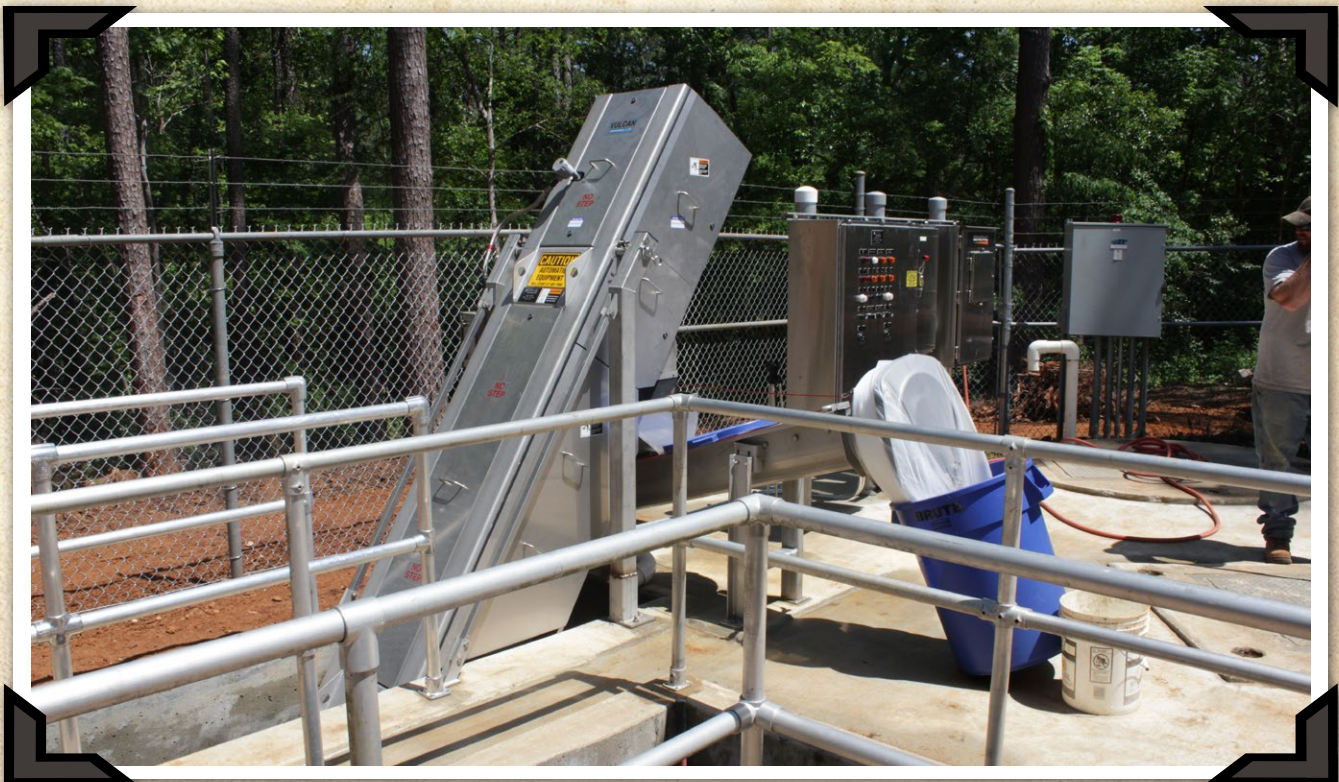
AUTOMATED BAR SCREEN LUFKIN STATE SUPPORTED LIVING CENTER LIFT STATION
