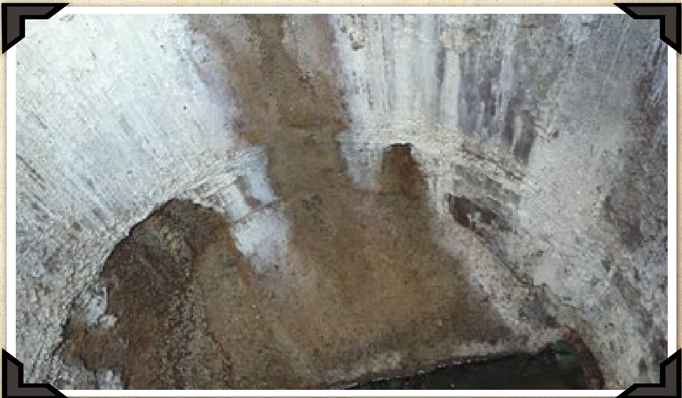
CALCIUM SULFATE FORMATION ON INTERNAL CONCRETE SURFACES IN MANHOLE
