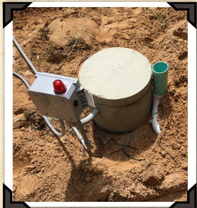
OSSF INSTALLATION INSPECTION
