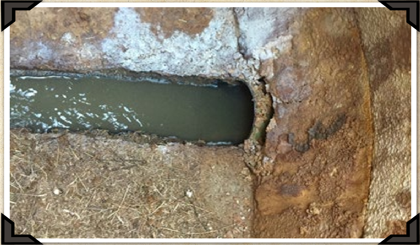
CORROSION INSIDE MANHOLE
