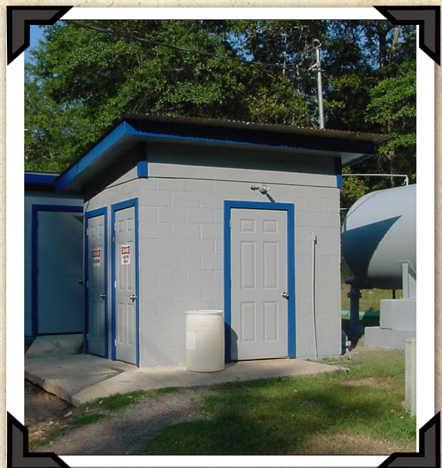
HOLMWOOD UTILITIES WELL #3 PUMP HOUSE
