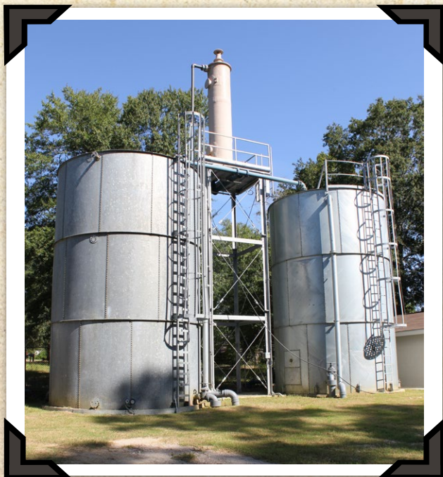
HOLMWOOD UTILITIES WELL #3
