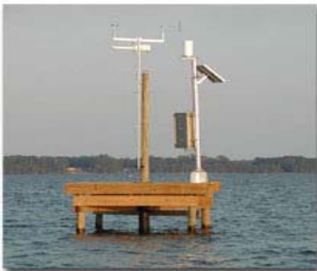
Caddo Lake in East Texas is home to two of the TCEQ's continuous monitoring platforms. The station collects data for weather and for water quality. On one pole are meteorological monitoring devices that measure for wind speed and direction and precipitation. Another pole holds solar panels to power the operation and a traffic box containing a data logger. All data is transmitted by radio. The water quality instrumentation is under water.
