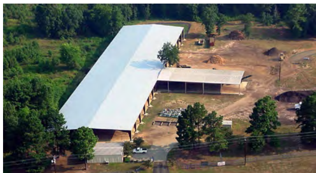
ANRA's Neches Compost Facility near Jacksonville
