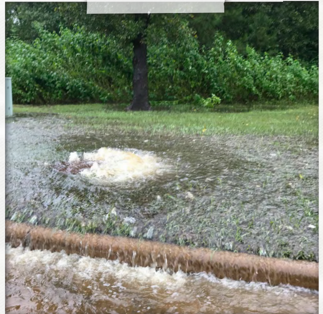
SANITARY SEWER OVERFLOW NEAR CEDAR CREEK AT ELLIS AUGUST 30, 2017
