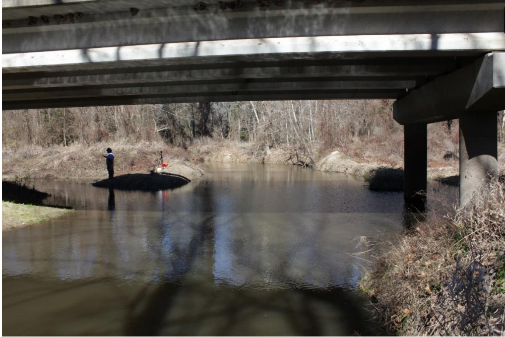
February 9, 2022: The most recent monitoring event at Piney Creek at FM 358 showed signs of continued damming, flooding, and litter accumulation in area, and accurate flow measurements are challenging to obtain due to these conditions.
