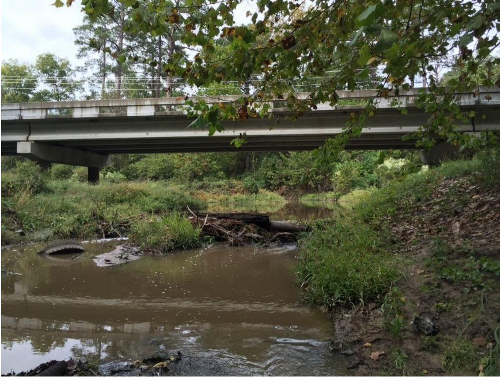
November 3, 2015: Brush and litter cause continuous damming, which prohibits steady stream flow.
