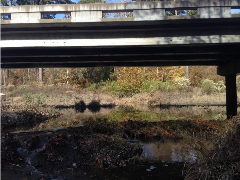
December 12, 2013: Water is present, but obvious damming has occurred.
