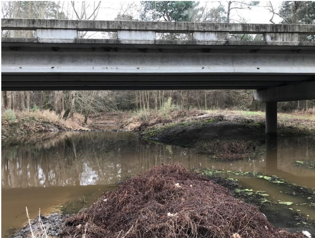
May 11, 2020: Damming prohibits normal flow, causing large areas of pooling beneath the bridge.
