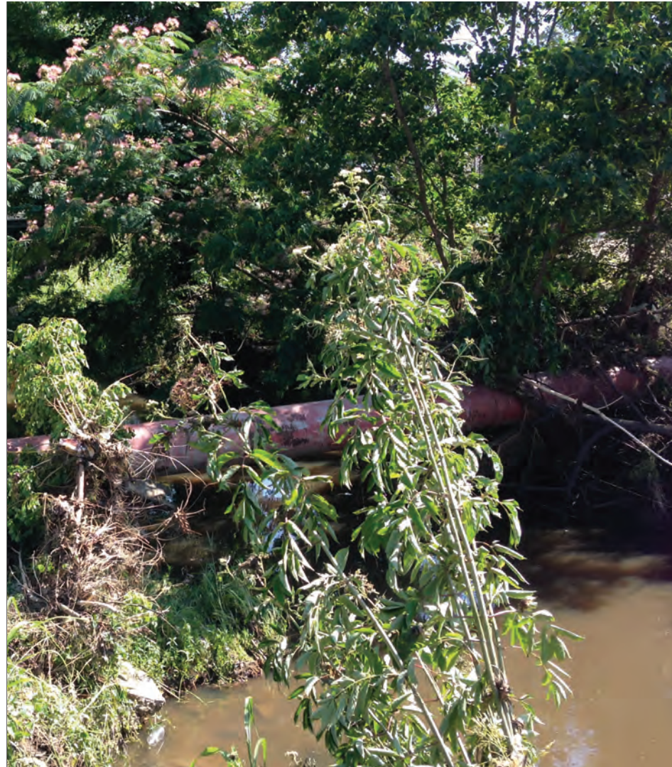
21434 - Cedar Creek at Ellis Avenue
