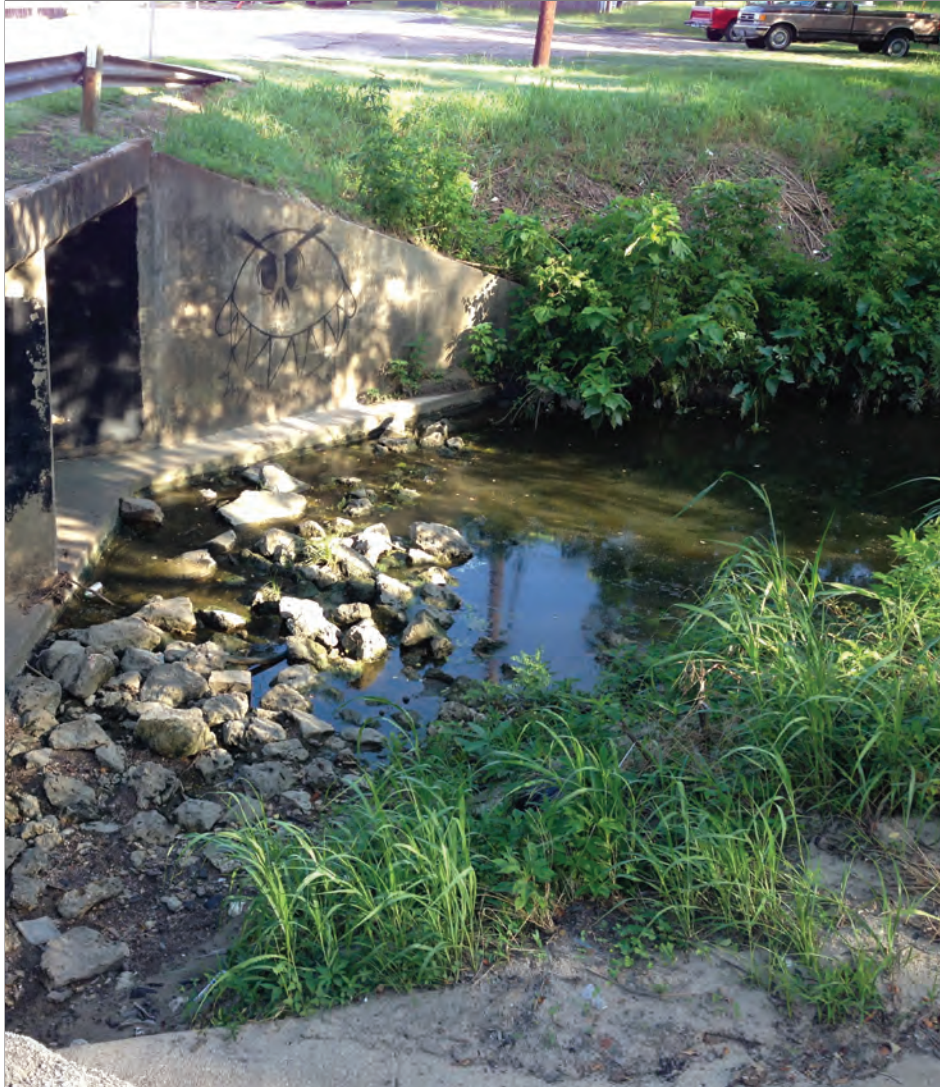
Bridge Crossing above 21433 - Hurricane Creek downstream of Kiwanis Park Drive
