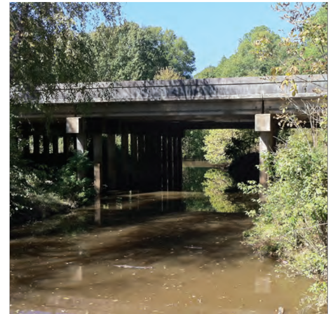
Bridge Crossing at 16076 - Attoyac Bayou at US 59
