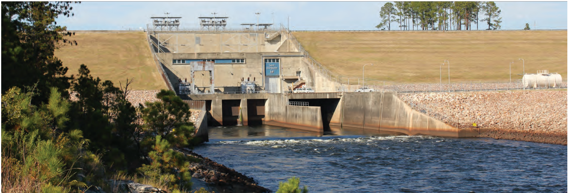
Spillway at Dam on Sam Rayburn Reservoir
