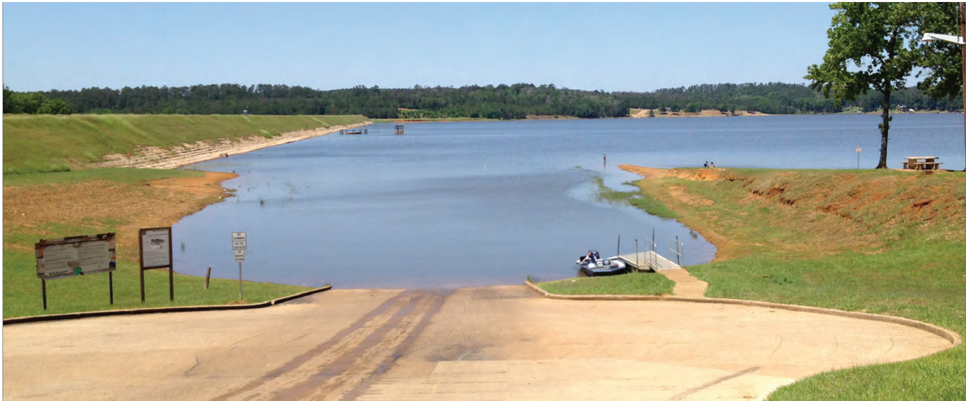
Boat Ramp near Station 15801 - Lake Nacogdoches At Dam
