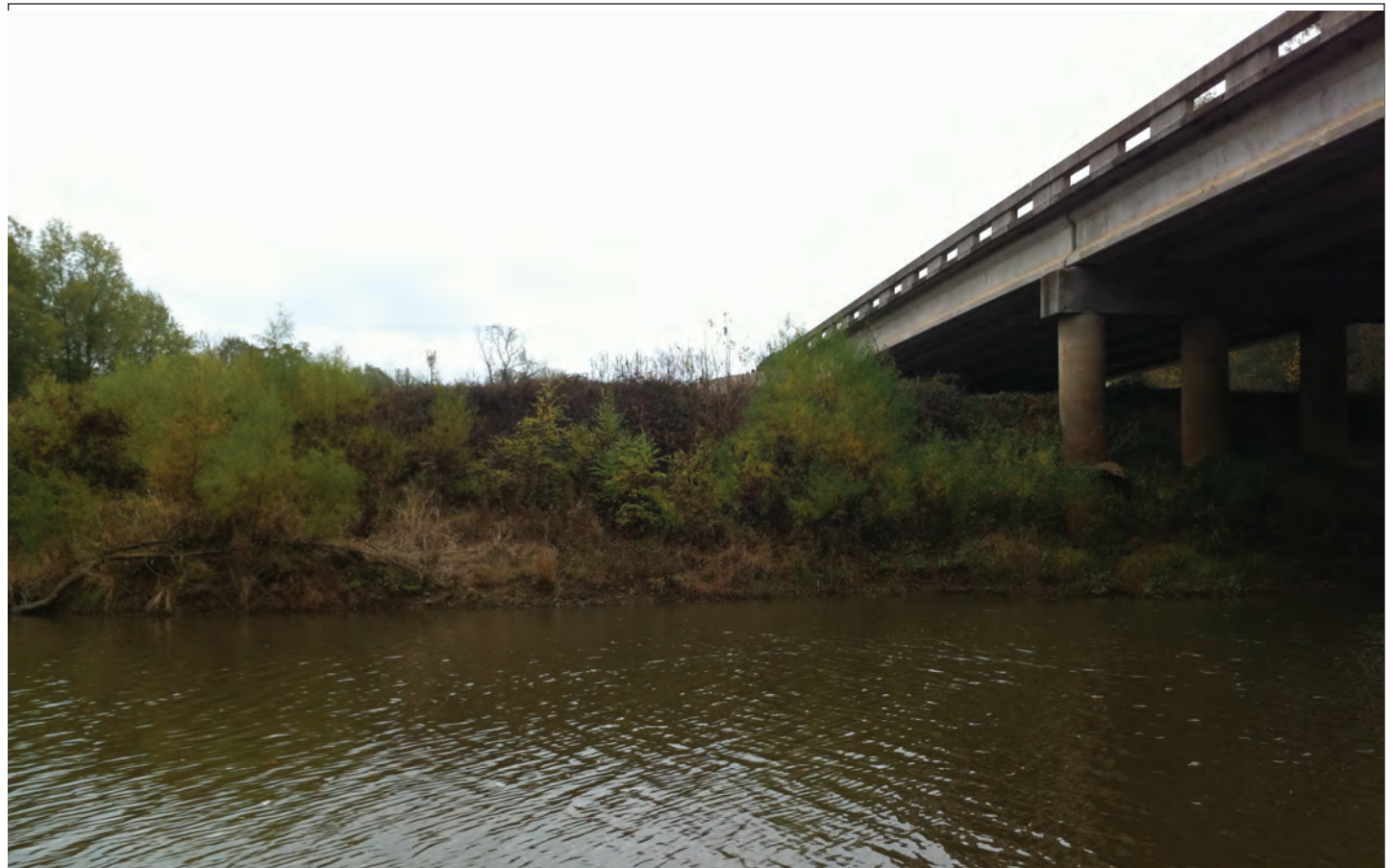
Bridge Crossing at Station 10630 - Angelina River at SH 21
