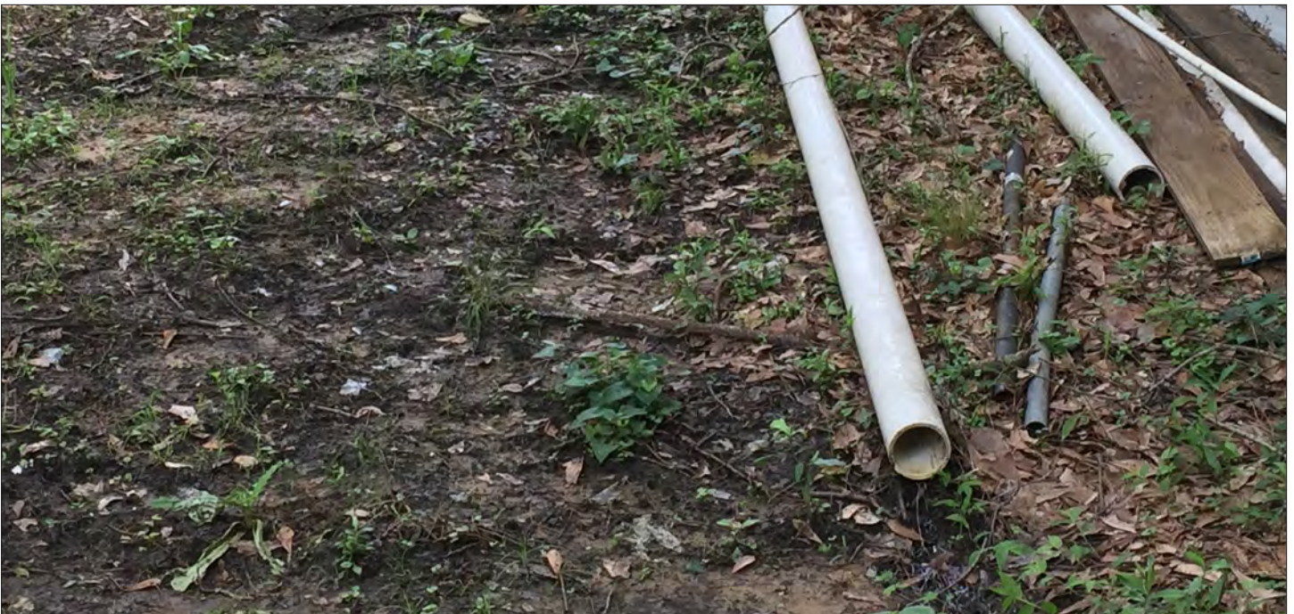
Site photographs of NAC-010 CM property prior to OSSF installation
