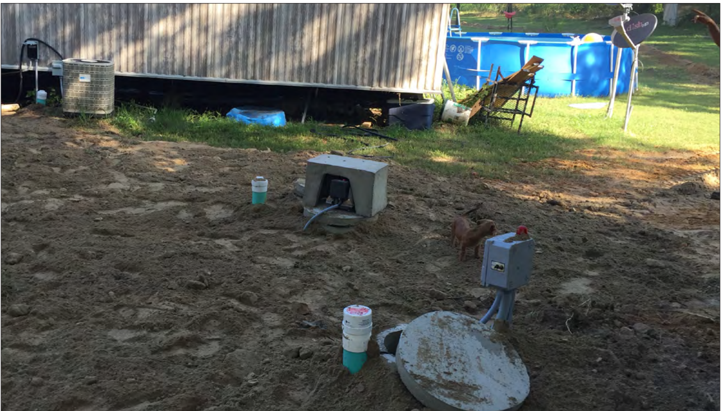
Site photograph of SA-001 BF property at inspection
