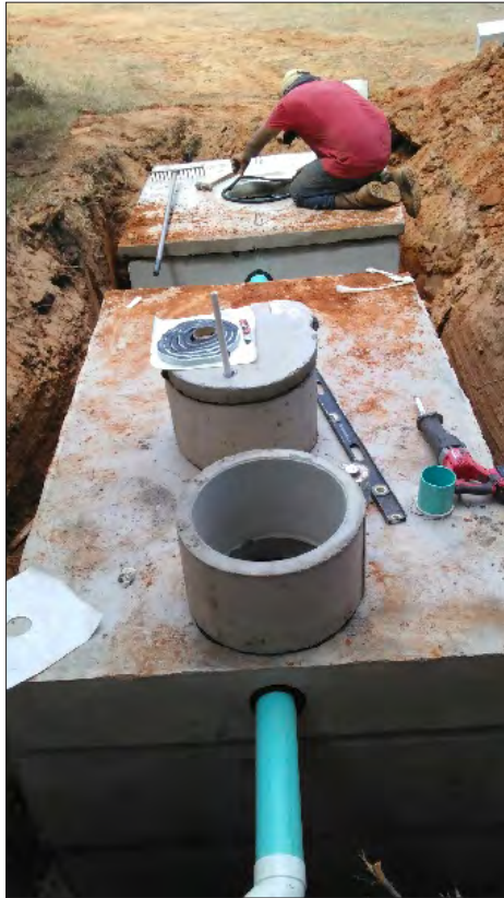
Site photographs of NAC-006 SM property during OSSF installation
