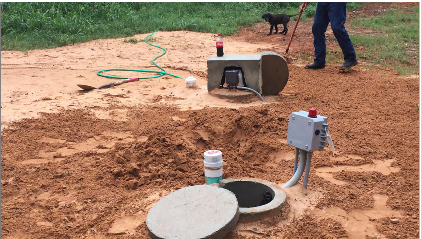
Site photograph of SH-001 JC property at inspection
