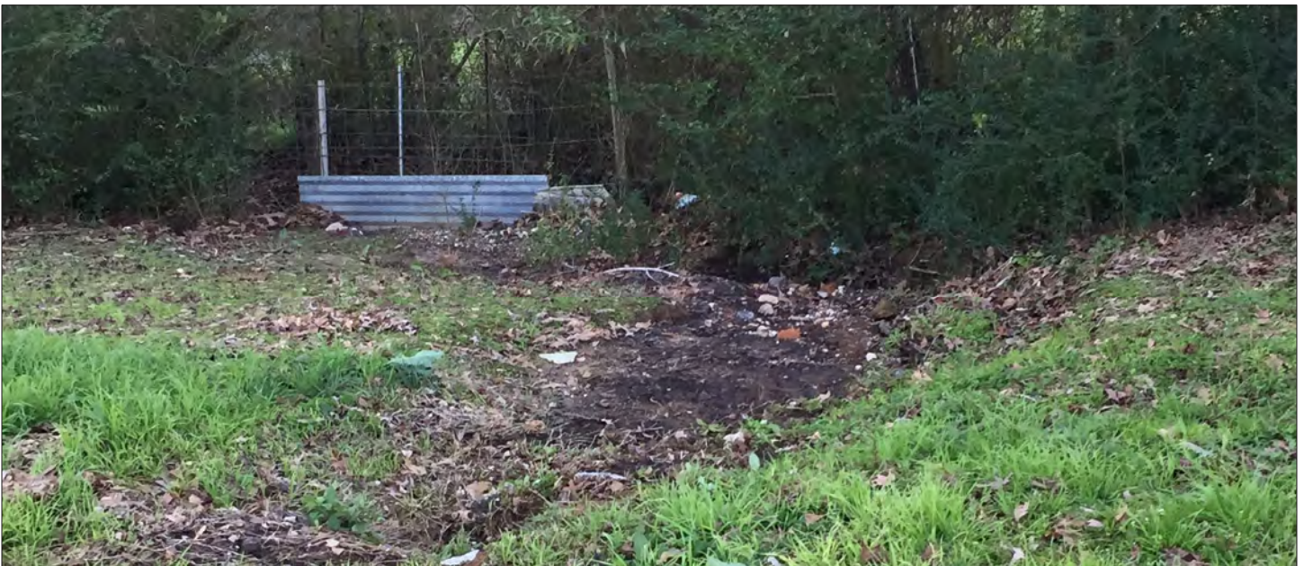
Site photographs of NAC-001 RT and NAC-002 RT property prior to installation
