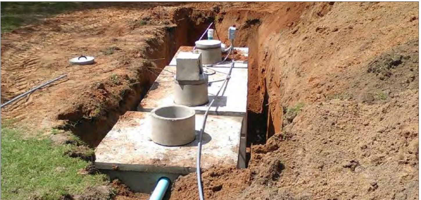
Site photographs of NAC-008 JP property during OSSF installation
