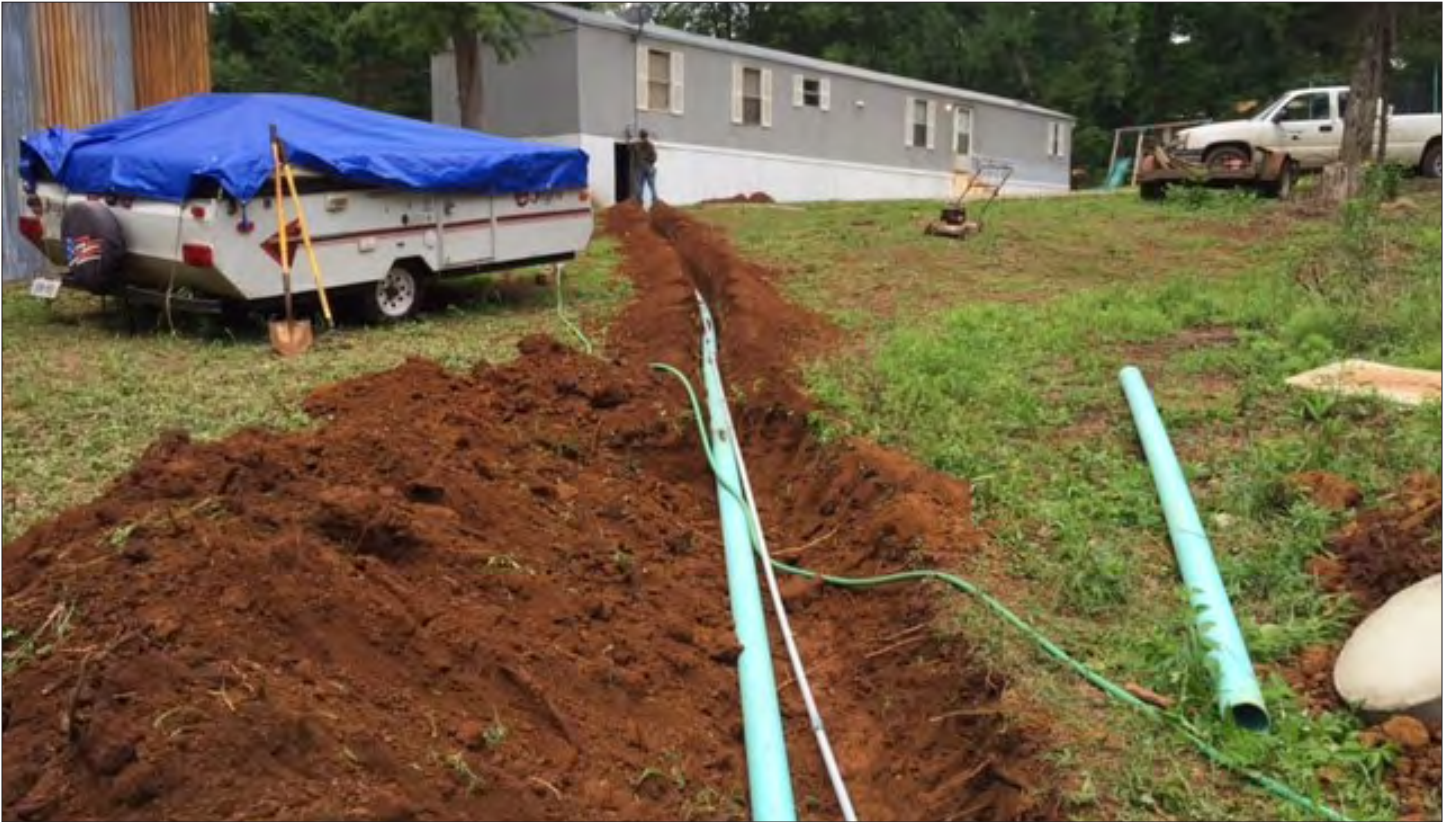
Site photograph of SA-008 JC property during OSSF installation
