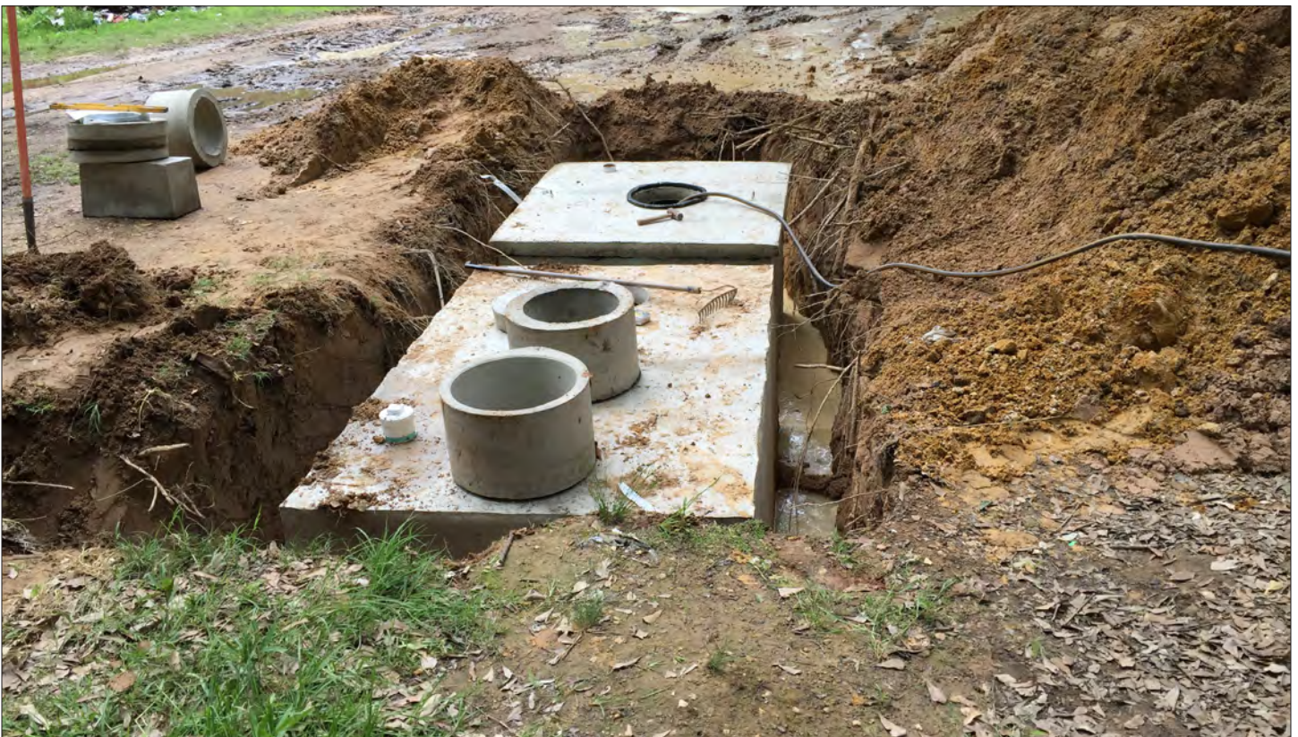
Site photograph of NAC-013 JE property at inspection
