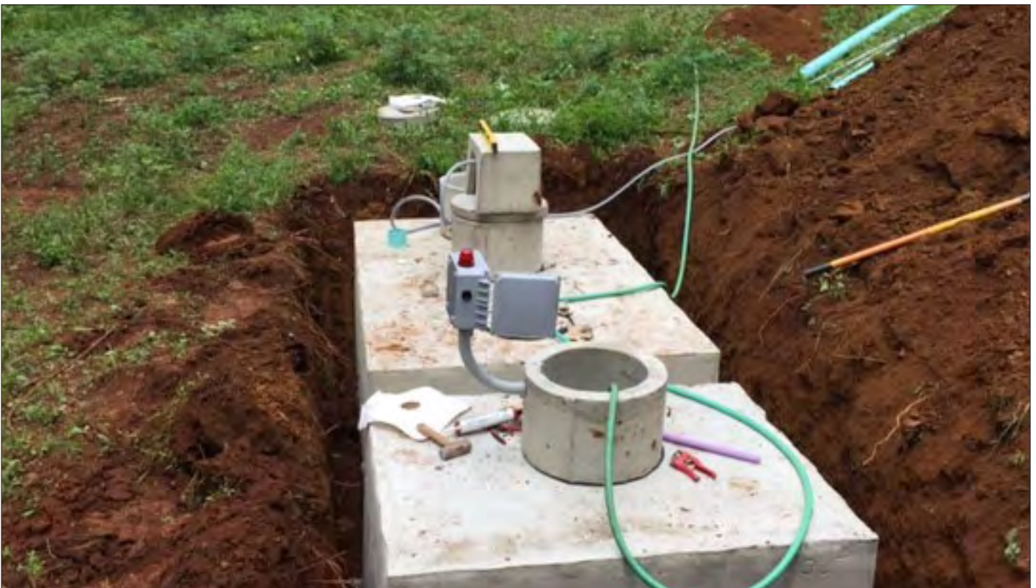
Site photograph of SA-008 JC property at inspection
