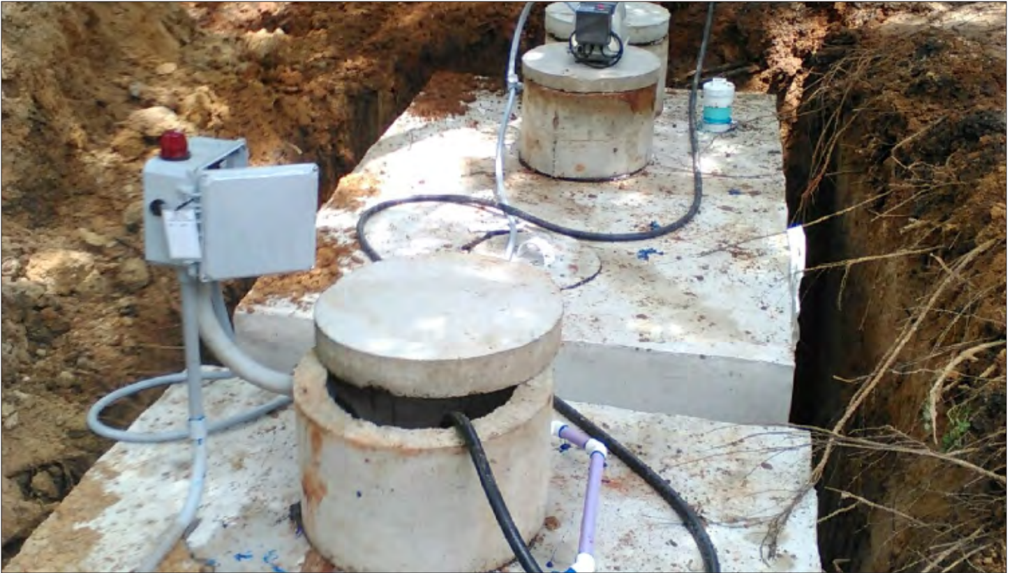
Site photograph of SH-002 CWC property during OSSF installation
