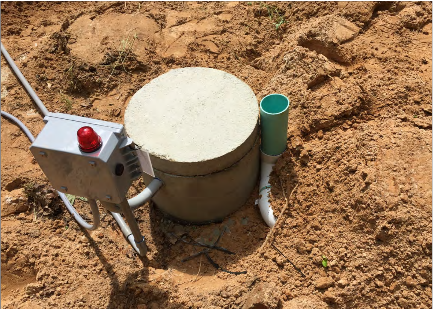
Site photograph of SA-002 KN property at inspection
