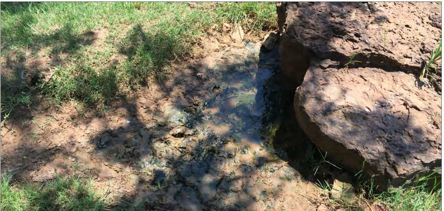
Site photographs of NAC-006 SM property prior to OSSF installation
