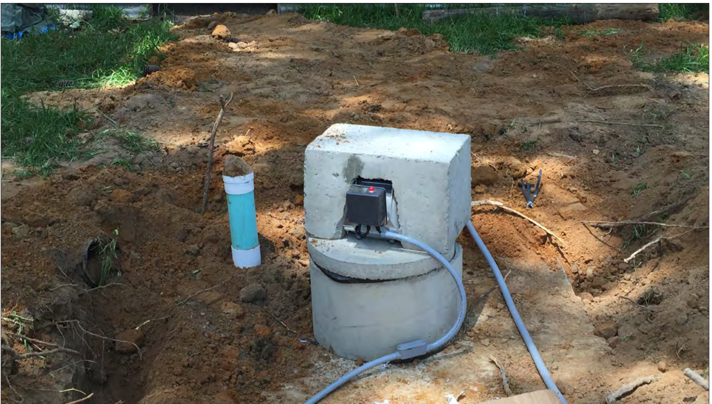
Site photograph of NAC-012 RE property at inspection
