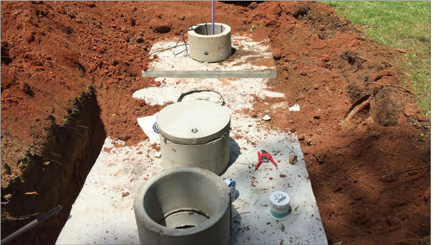
Site photographs of NAC-007 NC property during OSSF installation
