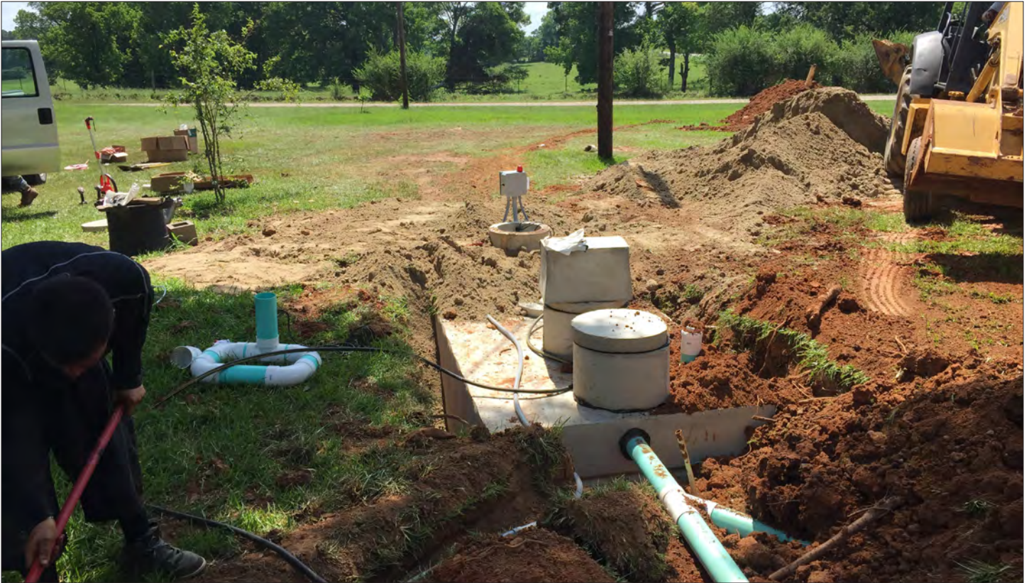
Site photographs of SA-006 DB property during OSSF installation
