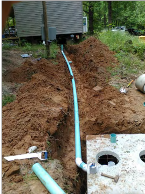
Site photographs of SA-002 KN property during OSSF installation
