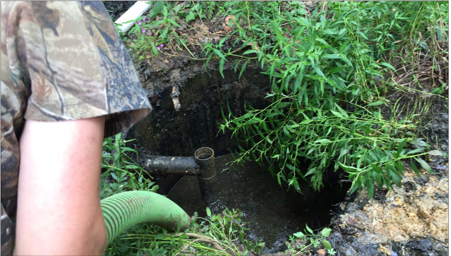
Site photograph of NAC-013 JE property during OSSF installation
