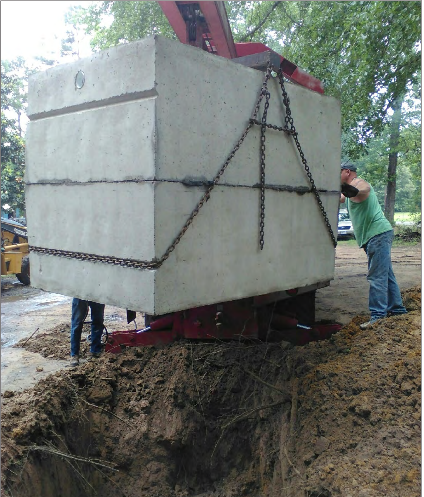
Site photograph of SA-003 IPL property during OSSF installation
