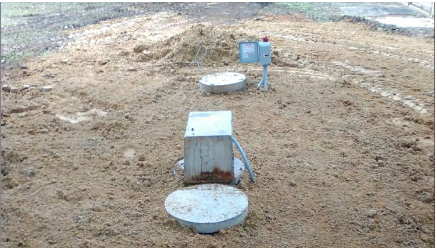
Site photograph of SH-002 CWC property at inspection
