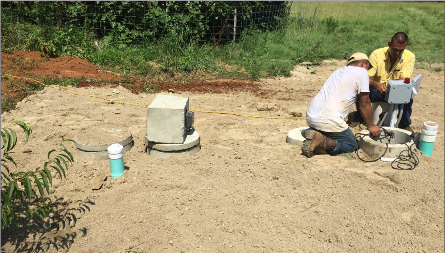
Site photograph of SA-005 EC property during OSSF installation
