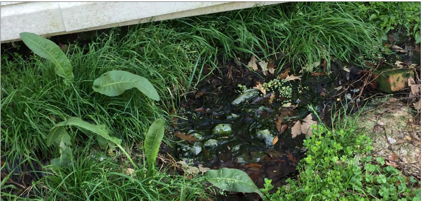
Site photographs of NAC-004 JDV property prior to OSSF installation
