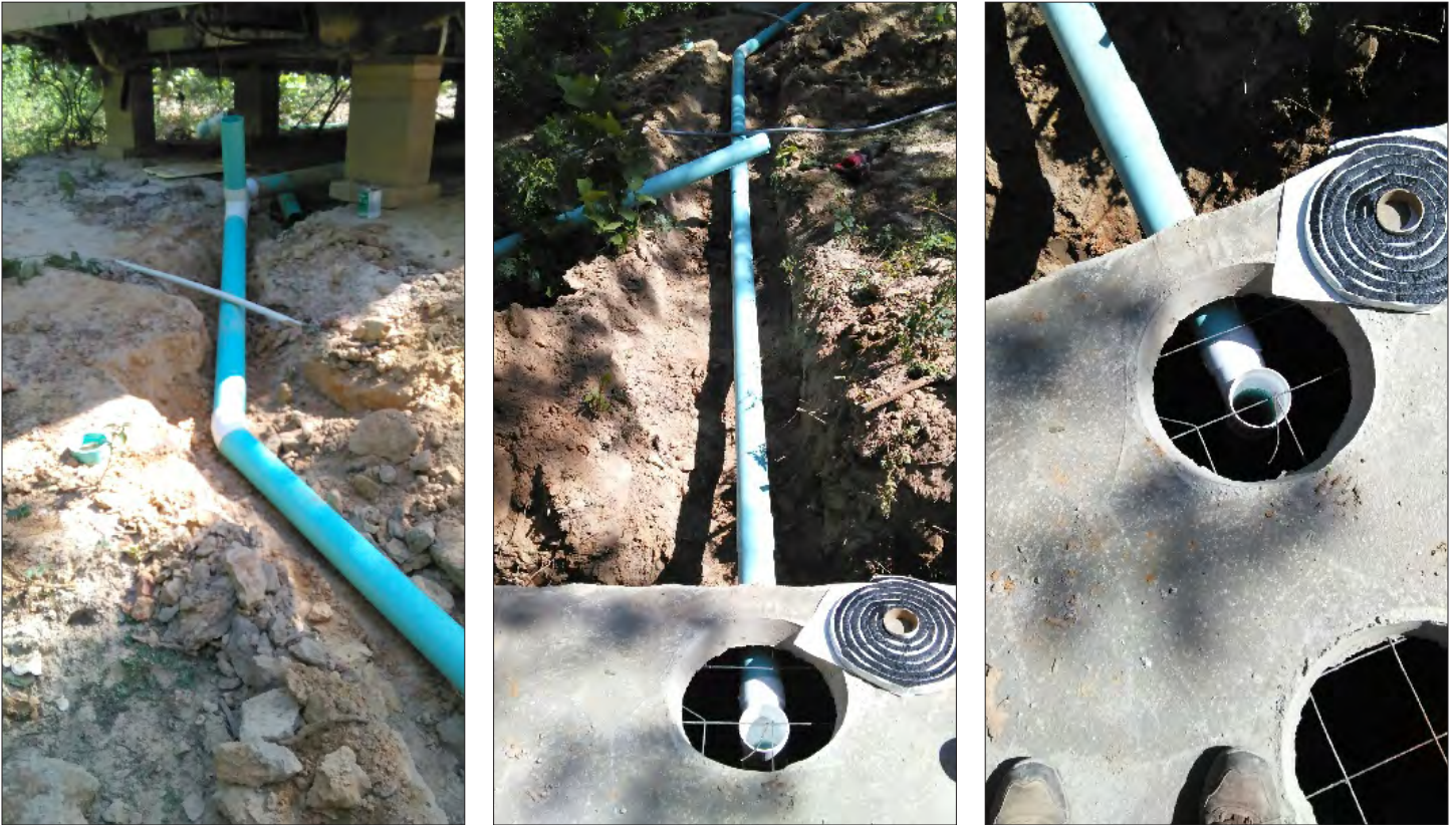
Site photographs of NAC-003 TG property during OSSF installation
