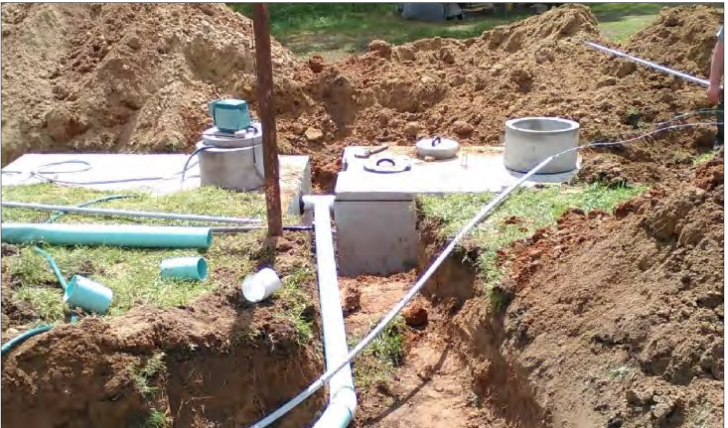
Site photographs of NAC-001 RT and NAC-002 RT property during installation
