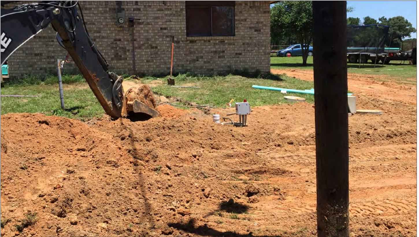
Site photograph of NAC-005 RG property during OSSF installation
