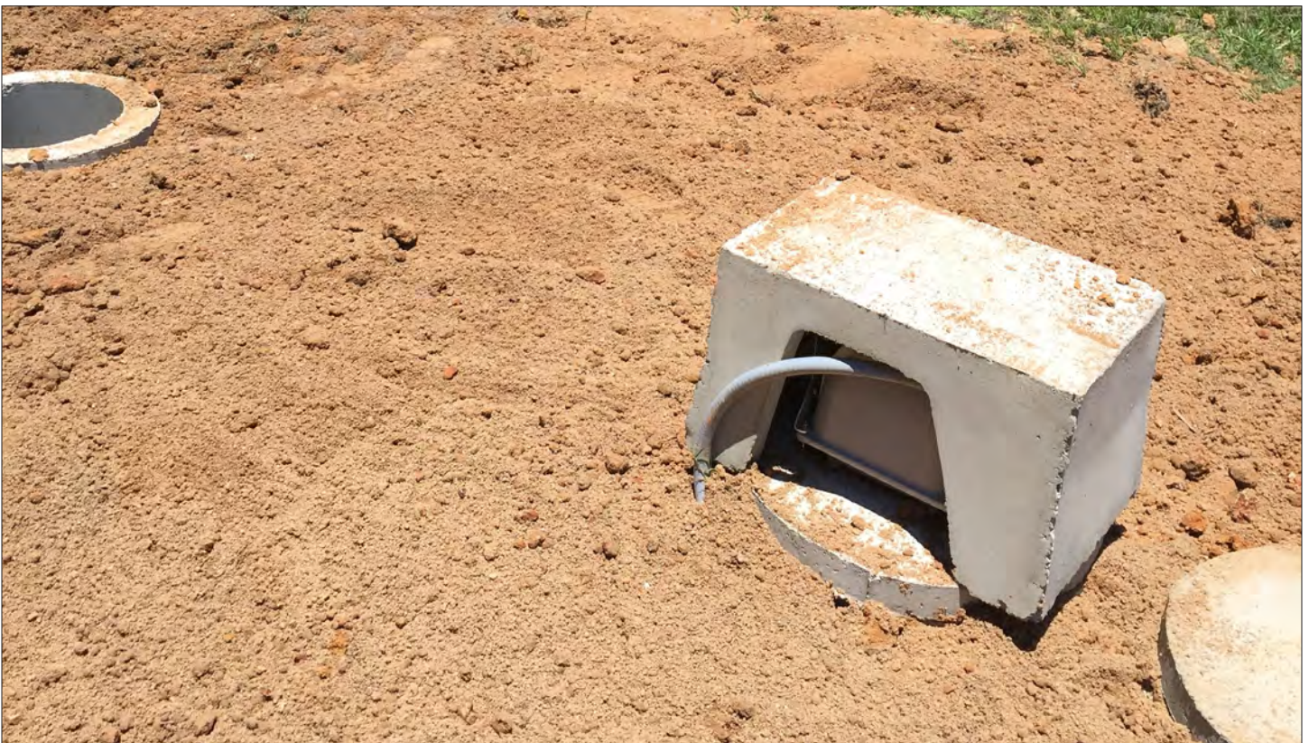
Site photograph of NAC-005 RG property at inspection
