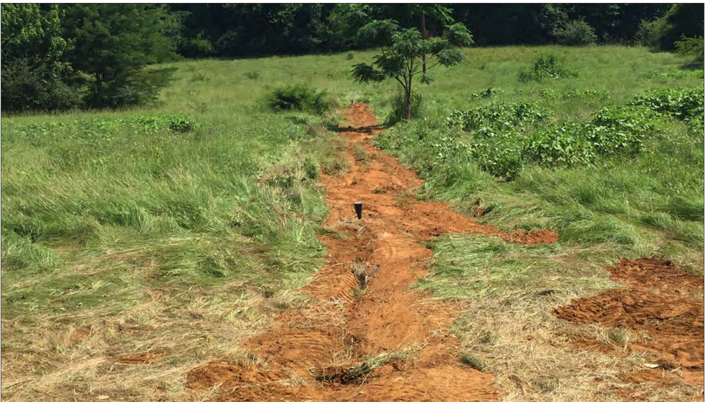
Site photograph of SA-005 EC property at inspection
