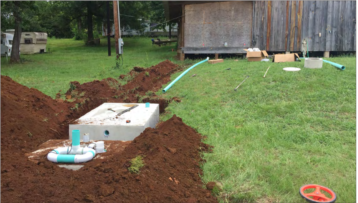
Site photographs of SA-007 KB property during OSSF installation
