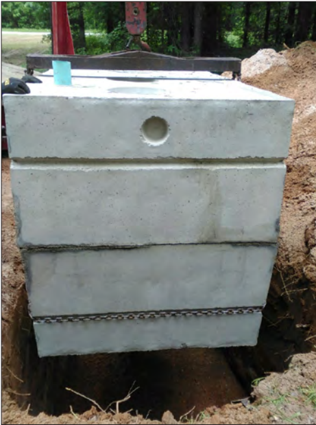
Site photographs of SA-002 KN property during OSSF installation
