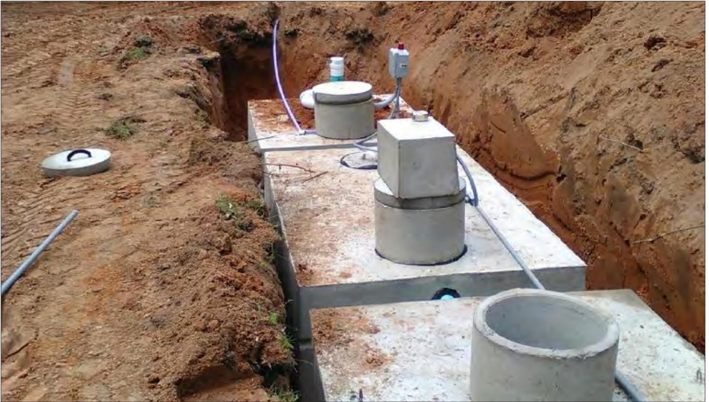
Site photograph of NAC-008 JP property during OSSF installation
