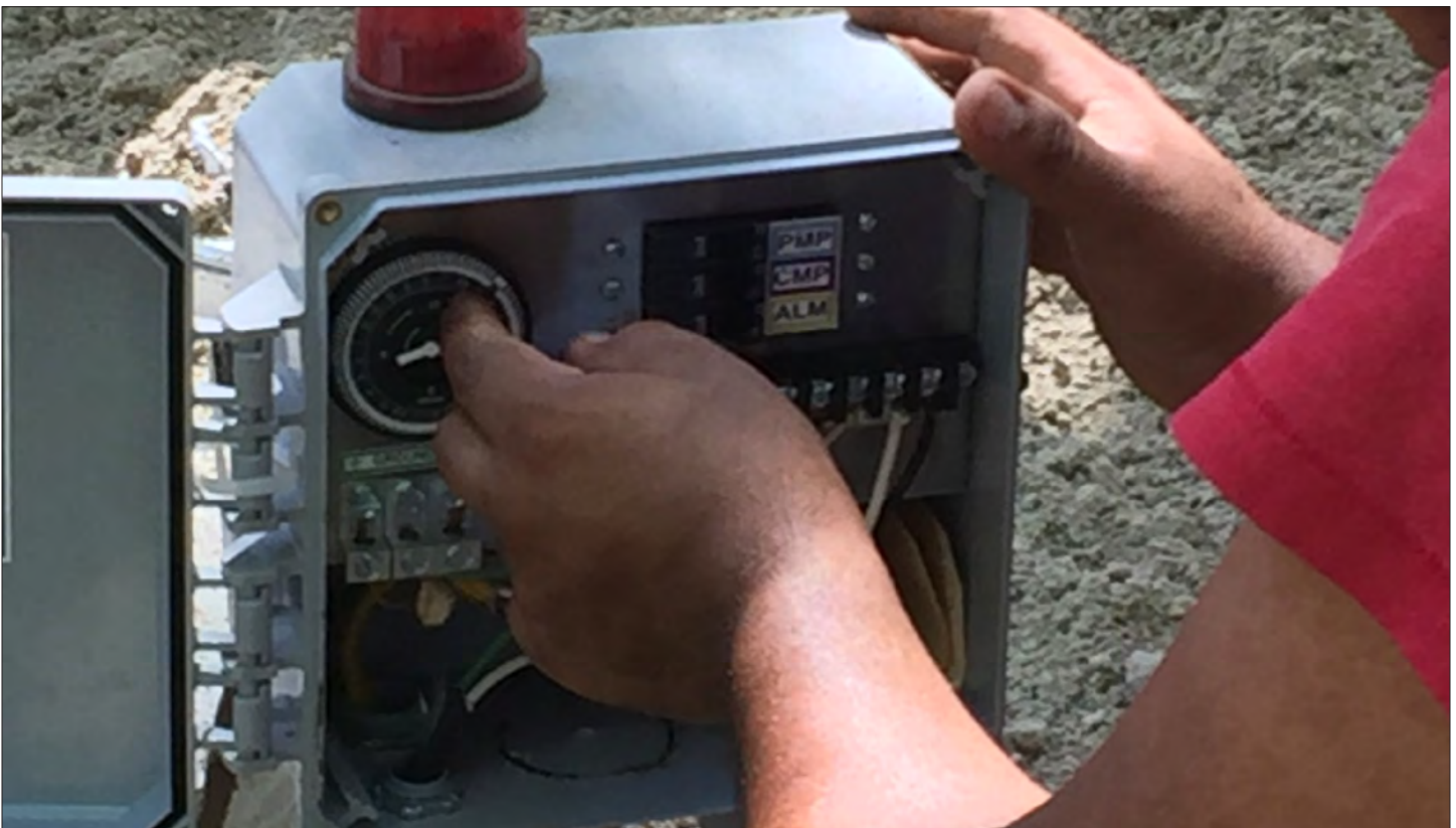
Site photograph of NAC-010 CM property at inspection
