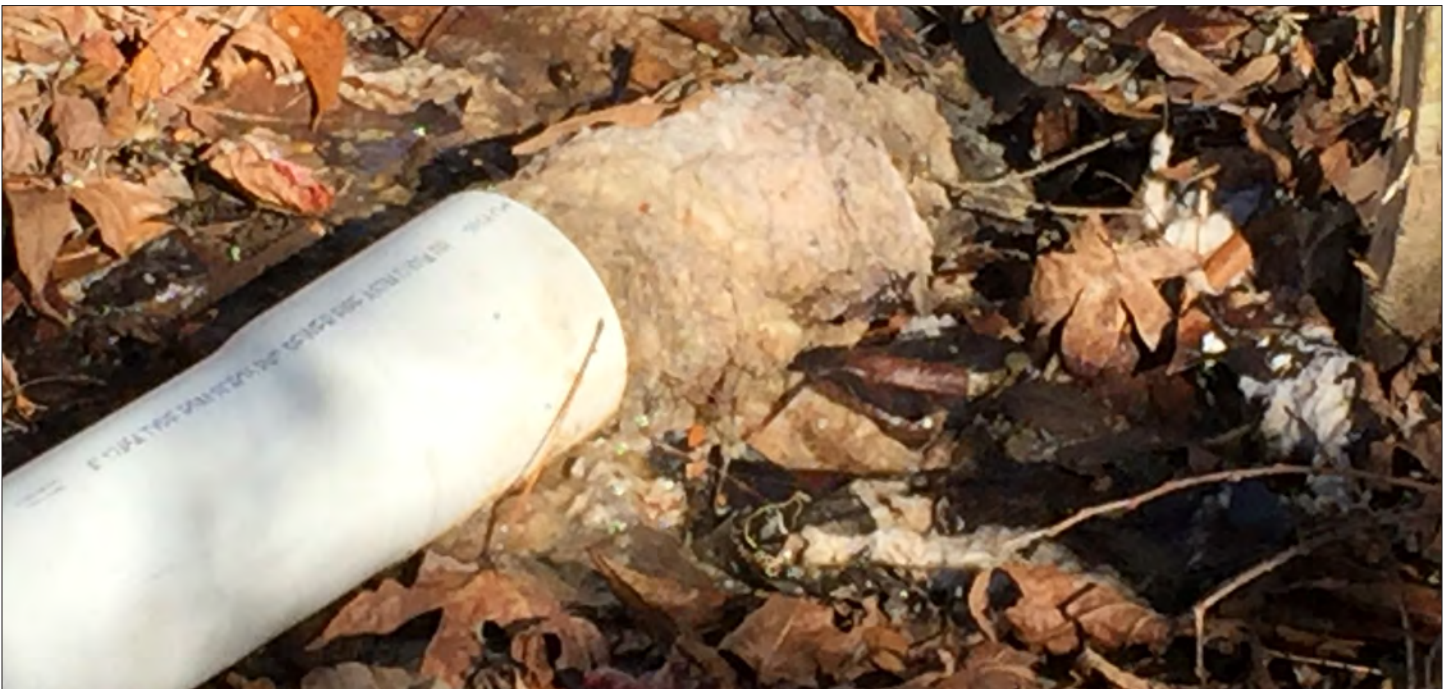
Site photographs of SA-002 KN property prior to OSSF installation
